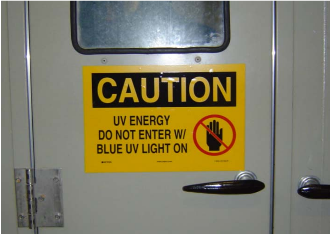
Figure 2.3: Typical warning sign for UVGI systems.
